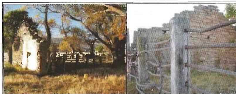
Above left, the end wall of the Nevis Crossing Hotel with cattle yards added on. Right, note the use of old mining hawsers in the fence.
